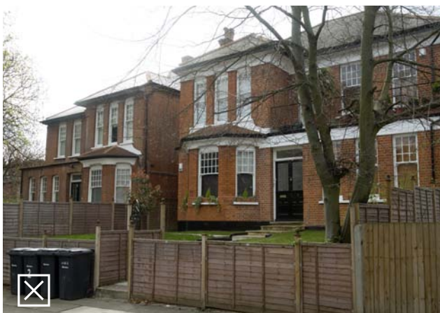
Fig 6.3: Unacceptable due to the poor quality of the boundary treatment
