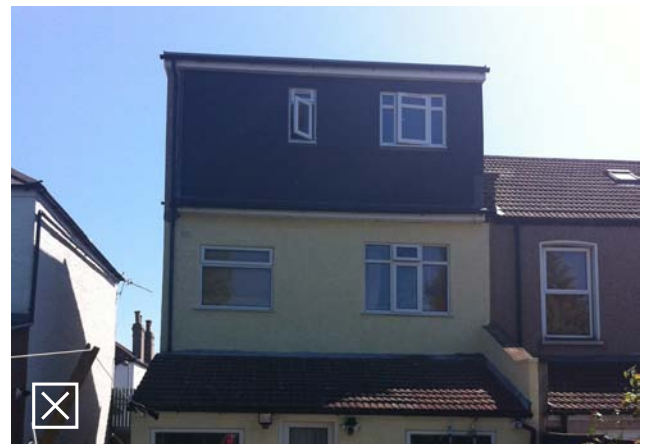
Fig 5.18: Unacceptable owing to the obtrusive nature of the extension. This obliterates the eaves, ridge or sides
