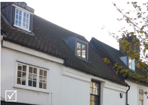
Fig 5.12: Acceptable example of dormer. They respect the proportions of the windows below and are an appropriate size
