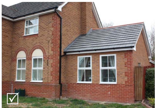
Fig 4.17: Sympathetic single storey side extension that steps back from original frontage.
