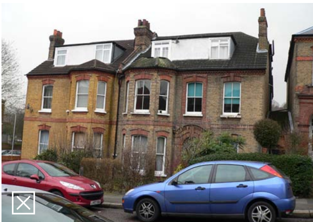
Fig 5.10: Unacceptable due to the dormers bulky nature and poor relationship with the elevation below
