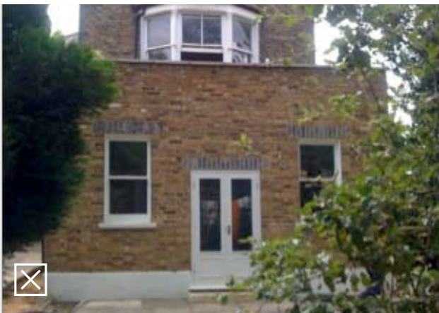
Fig 4.5: Unacceptable because the single storey rear extension is incongruous. This negatively impacts on the integrity of the original building form because it is too high, impacting on the first floor rear bay window
