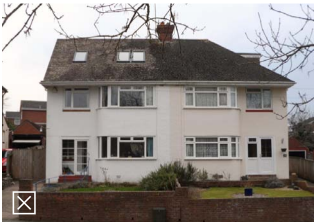
Fig 5.23: Unacceptable - Hip to gable extension is not permitted on a pair of semi-detached houses
