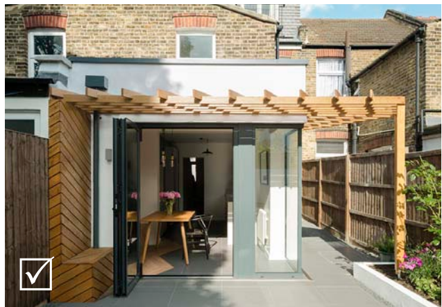
Fig 4.6: The extension clearly disguises itself from the host building and has a positive relationship with neighbouring properties
