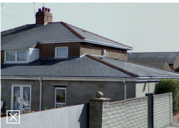
Fig 4.2: Unacceptable because the wrap around extension overwhelms the original dwelling and impacts on the first floor windows.
