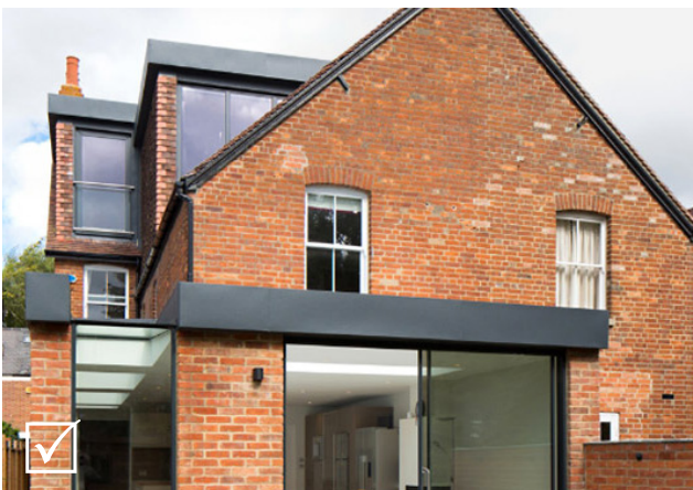
Fig 5.27: Acceptable due to sympathetic materials and they are both set in from the original roofline
