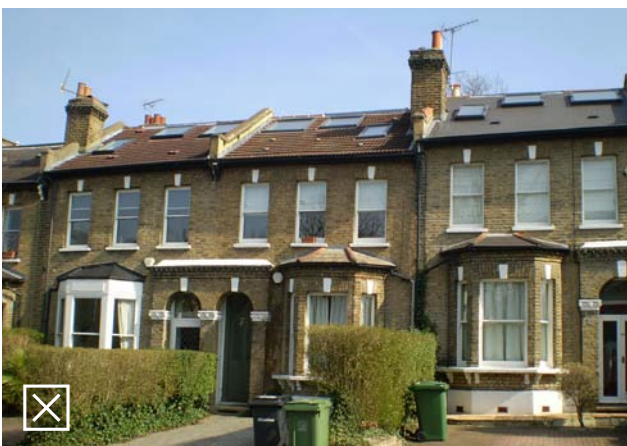
Fig 5.4: Unacceptable due to irregular roof light sizes and positioning
